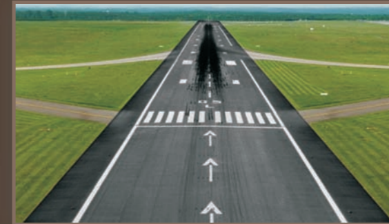
Airport Striping & Paving
